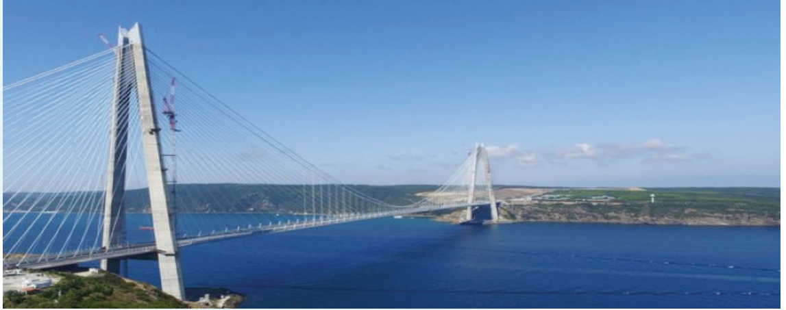
Yavuz Sultan Selim Bridge is the widest suspension bridge in the world with a width of 59 meters and the longest spanning one that has a rail system on it, with a main span of 1408 meters. Another first of the bridge is that it is the suspension bridge with the highest tower of the world, with a height of more than 322 meters.
