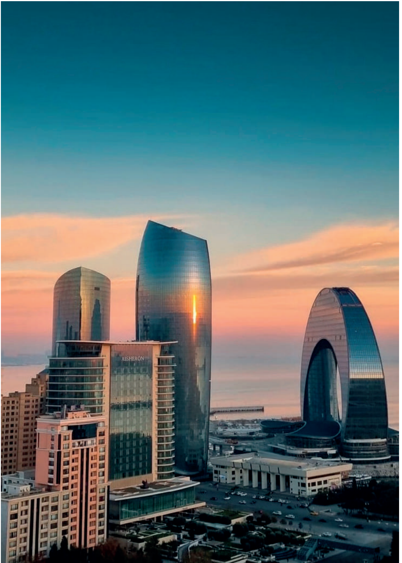
The Crescent Development Project, implemented by Pasha Real Estate, comprises three key buildings: Crescent Mall, Crescent Residence, and the City Tower office building. The project's standout feature is the adoption of advanced technologies, such as the Sea Water Cooling System.
